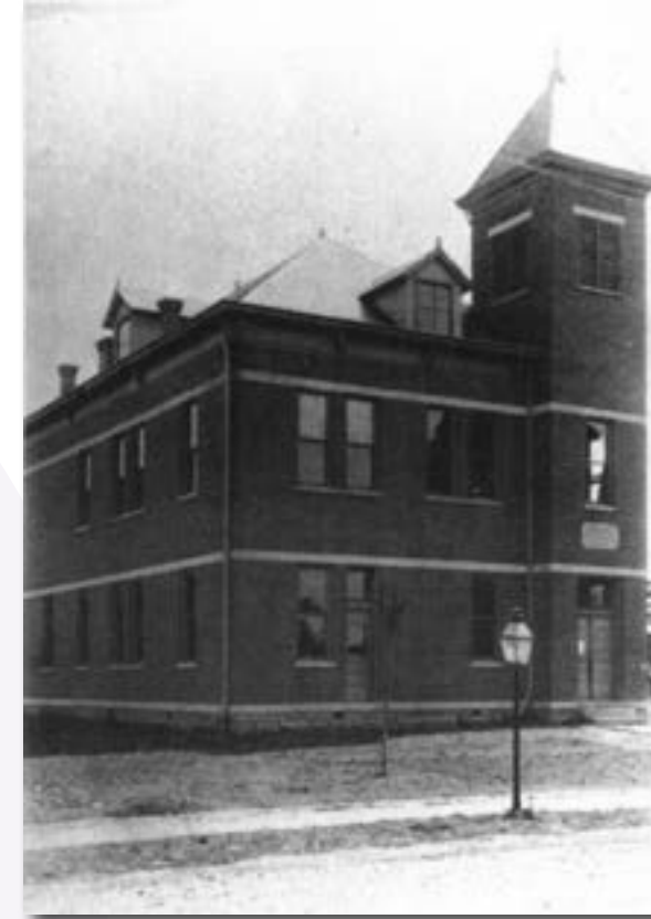
Glandorf Village Hall, built in 1901 and razed in the late 1960s.
